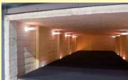
Furnace chamber with eight high-speed burners
