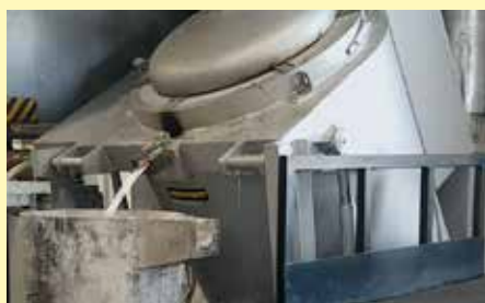
Tilting furnace KBR 240/11 during filling of a transport ladle
